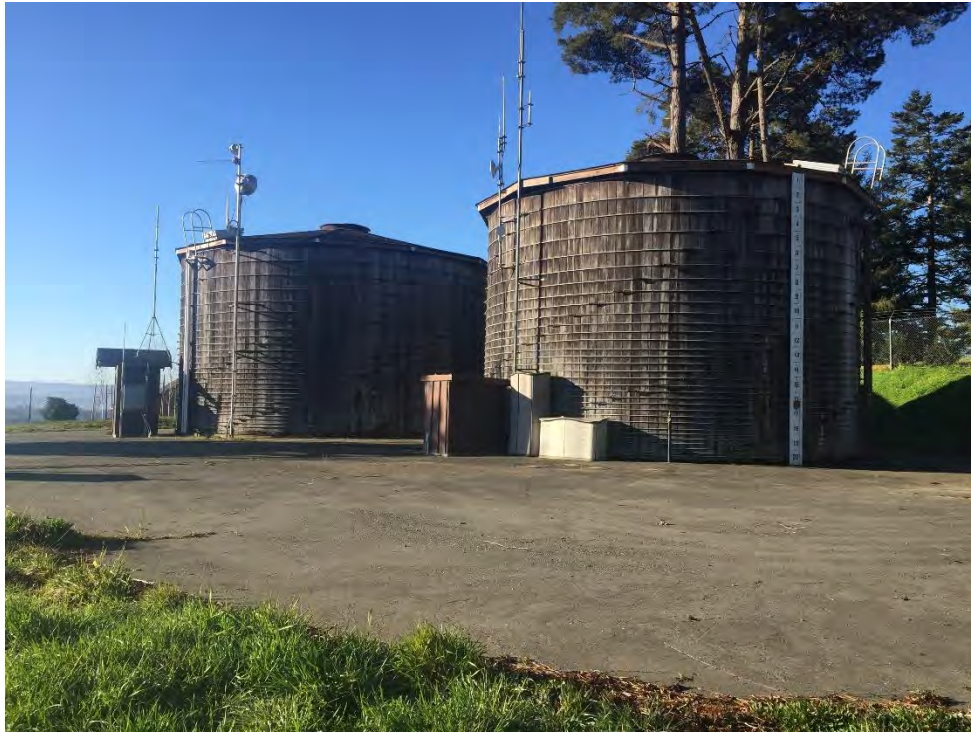
Photo 1 - View of Site facing northwest, both existing redwood tanks
