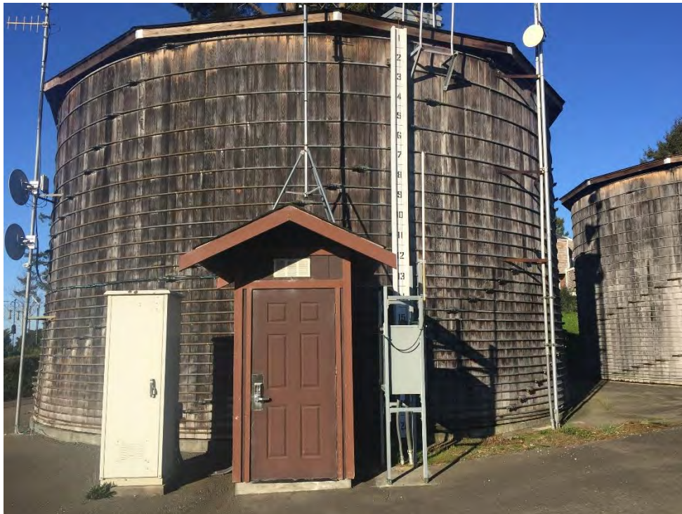
Photo 2 - View of Site facing south north, existing 150,000-gallon redwood tank
