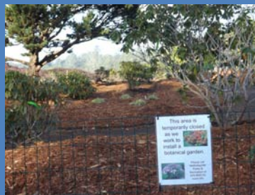
Installing of the Botanical Garden
