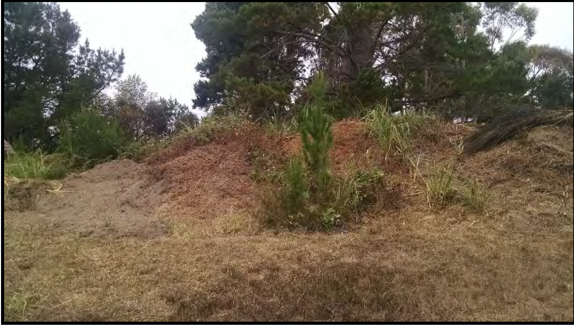
Figure 14. Detail of project area showing degree of vegetal growth on push pile. View north, September 9, 2021.
